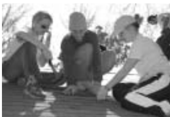
Left: Volunteers at work during a recent Saturday. Photo by Hiro Motegi. Photos on Feb. 2005 Impact cover also by Motegi
